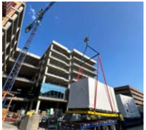
August 9, 2025 - 1501 Lavaca air handler units being flown to the appropriate floor.
